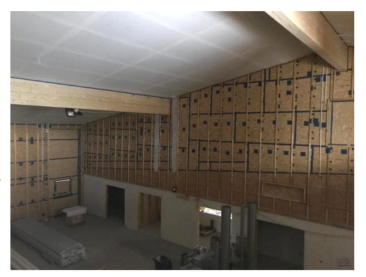
Boarding was used internally utilising airtight tape on all joints.
