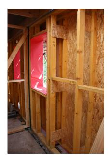
The Larsen truss system allows for a thicker wall space. This space was filled with Warmcel Insulation.
