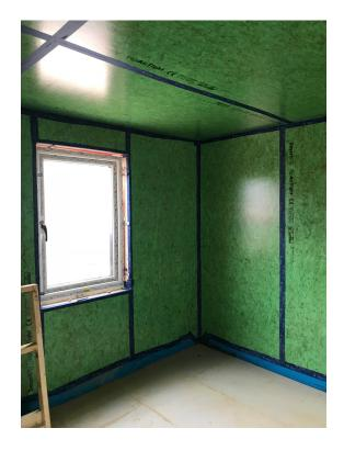
Smart ply airtight boarding was used internally utilising airtight tape on all joints.
